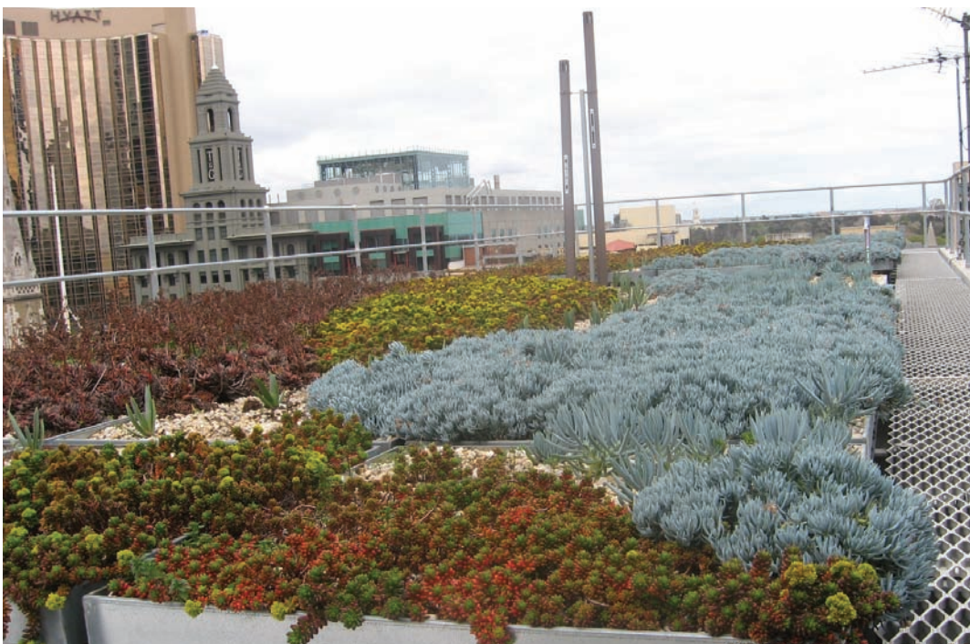
Melbourne City Council's CH 2 building in central Melbourne features an energy-saving rooftop garden.
